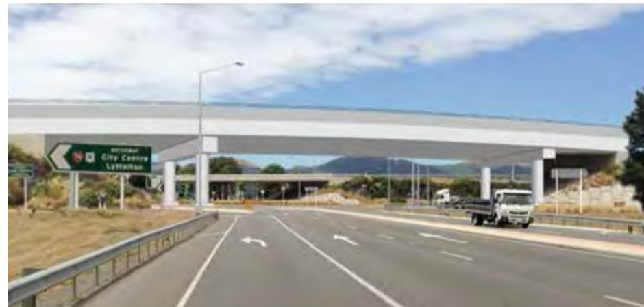
The new overbridge joins Wigram Road and Magdala Place, better connecting the south-west of the city with Riccarton and Addington.
