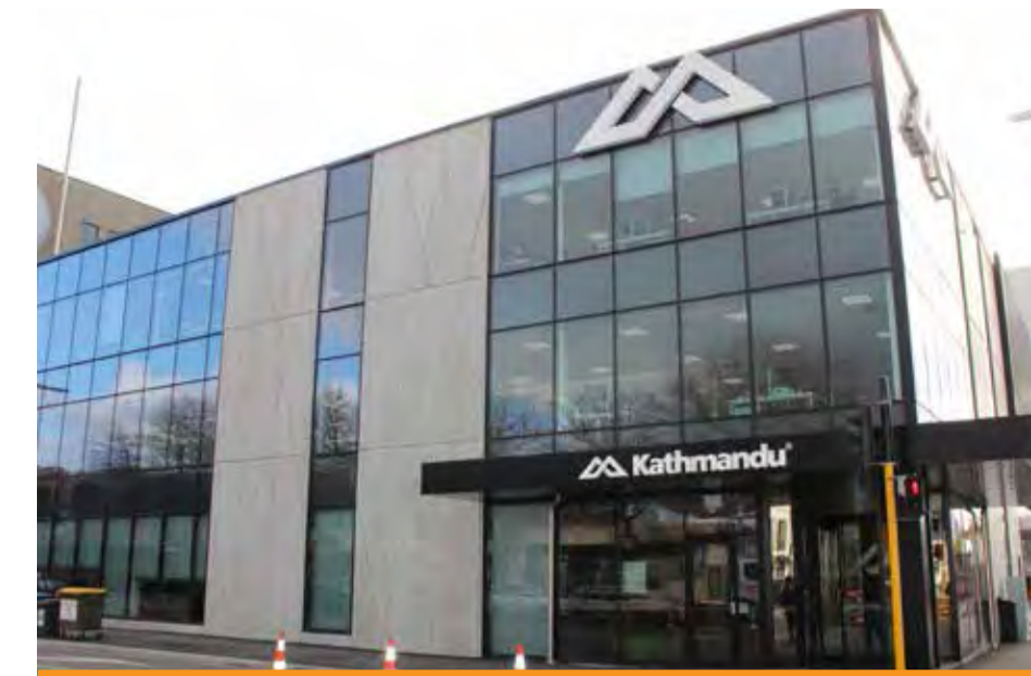
Floors made from recycled rubber tyres and timber from earthquake-damaged buildings were used in the new Kathmandu global headquarters.
