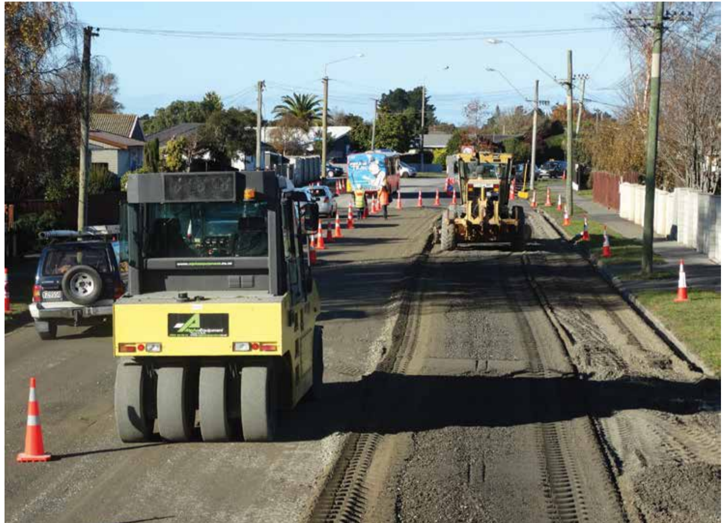
Repair of Mairehau Road in Parklands.
