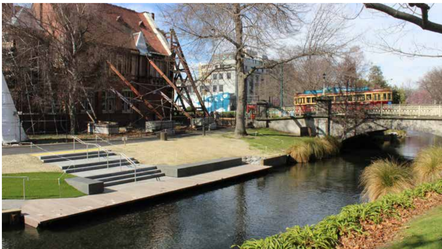
The Worcester Bridge punt stop (with wheelchair access ramp) provides an attractive access point to the water and a new home for aquatic life.
