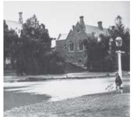
Avon Provincial Chambers shown in flood in 1868.
