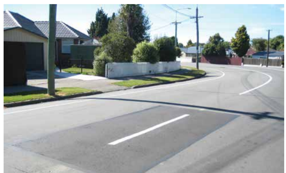
An example of patch repair on Clyde Road in Ilam.
